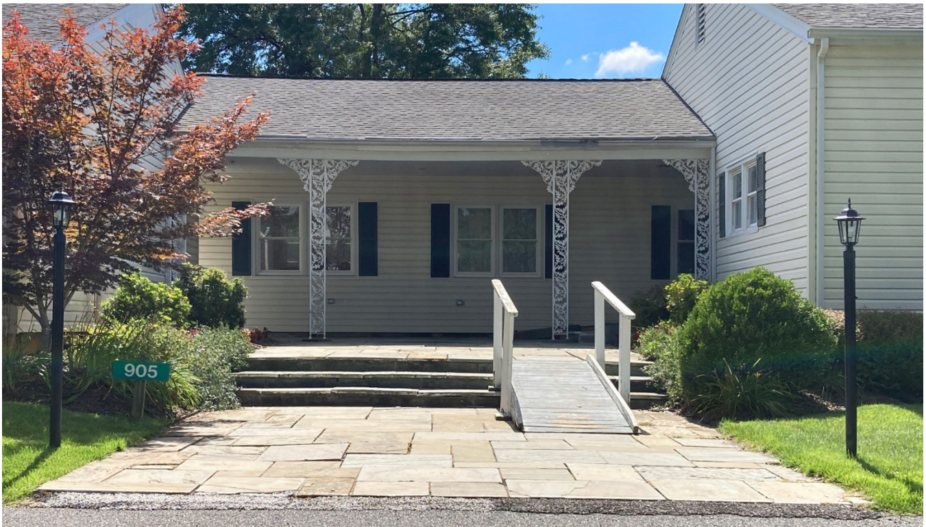
Entrance patio and steps scheduled for replacement, October 23 through November 8
